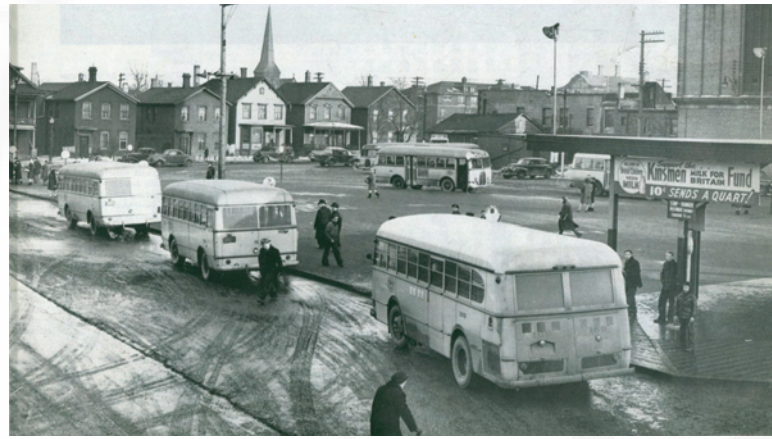
The downtown S.W.A bus depot in 1940. These buses replaced the streetcars. In Reflections of Windsor .
